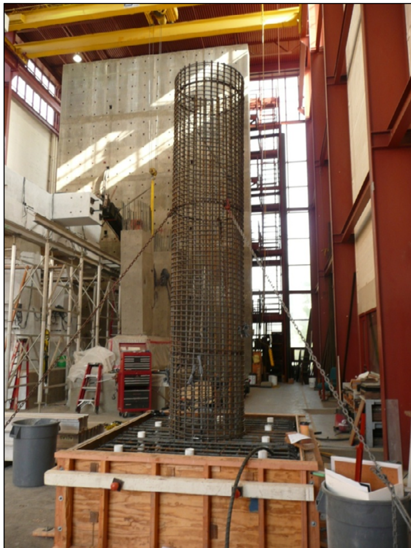
Figure 5.2: Completed Column and Footing Cage
