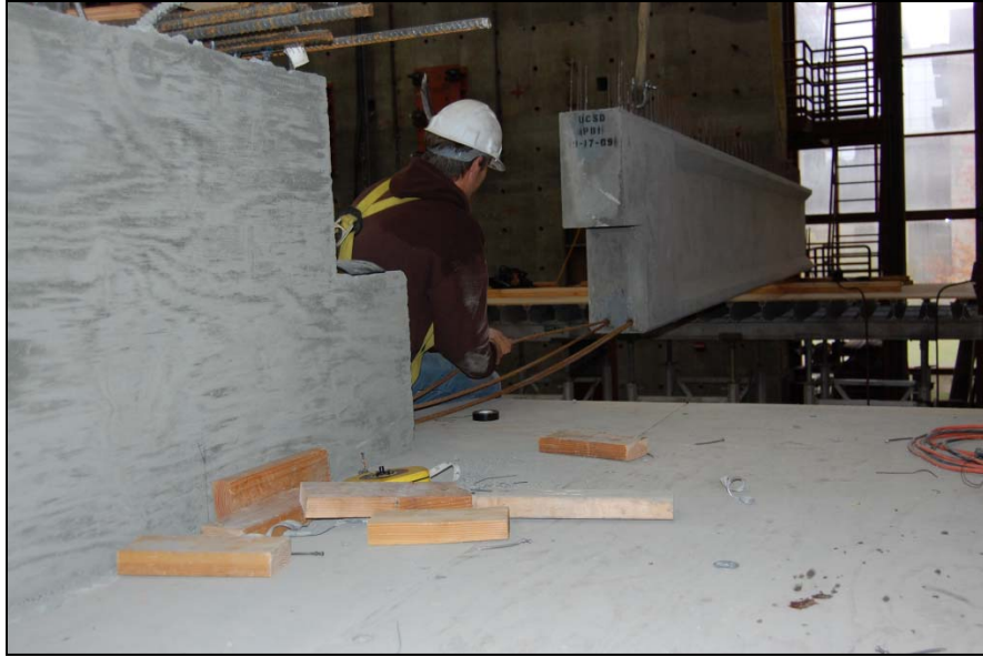
Figure 5.11: Pushing the Strands through the Girder
