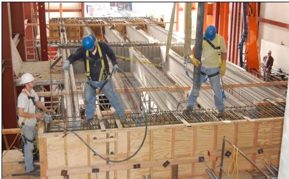
Figure 5.6: Casting of the North Abutment
