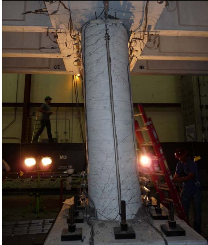
Figure 6.1: A Close-Up View of the Column Performance at +7.0 in. of Lateral Displacement ( \mu_{\Delta}=+10 )
