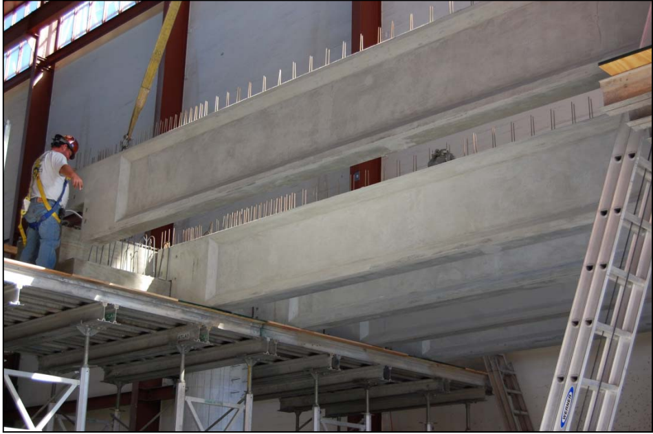
Figure 5.5: Installation of Southern Girders
