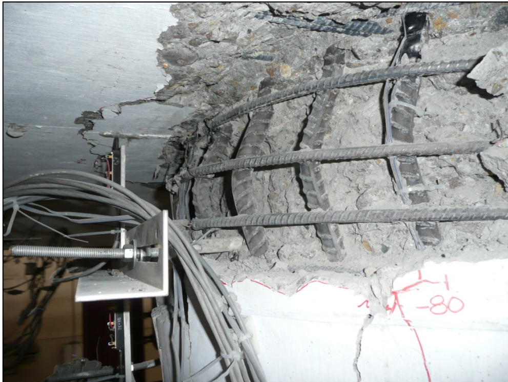
Figure 6.3: Buckling in the Top Column Hinge on the North Side at \mu_{\Delta}=10
