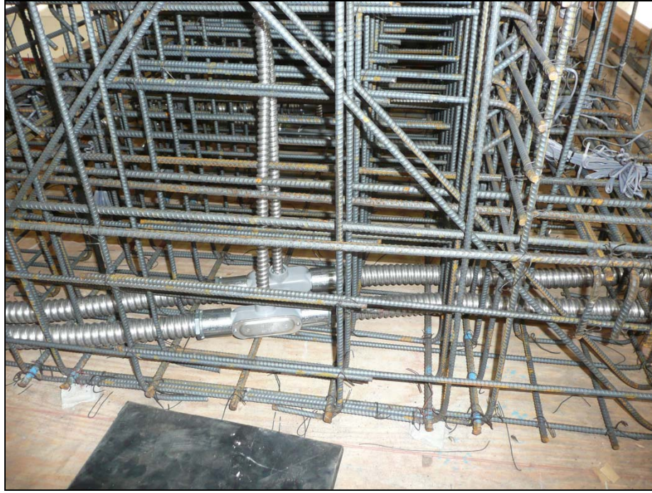
Figure 5.9: Routing of Bent Cap Ducts
