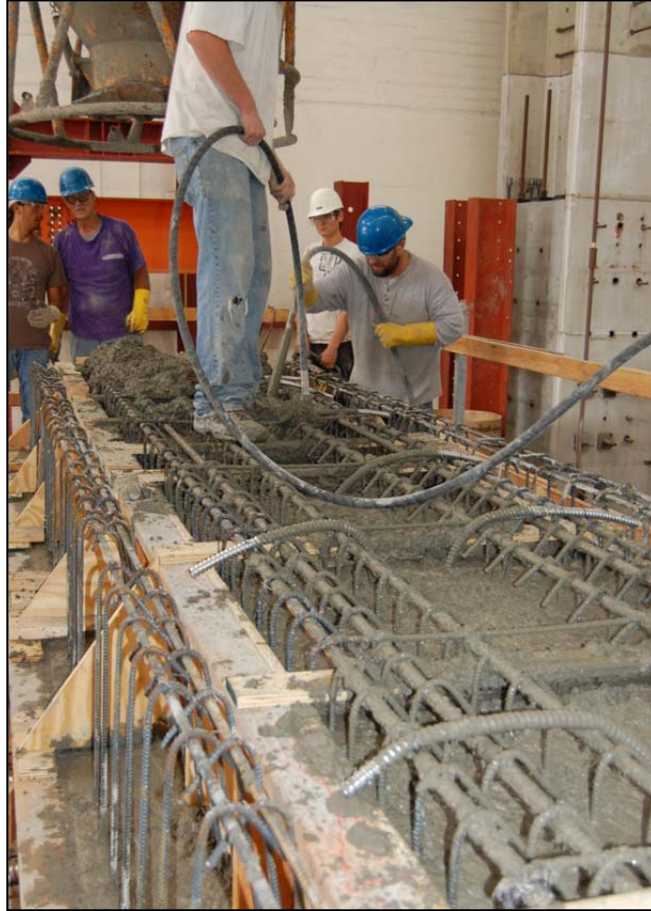
Figure 5.8: Casting of the Bent Cap
