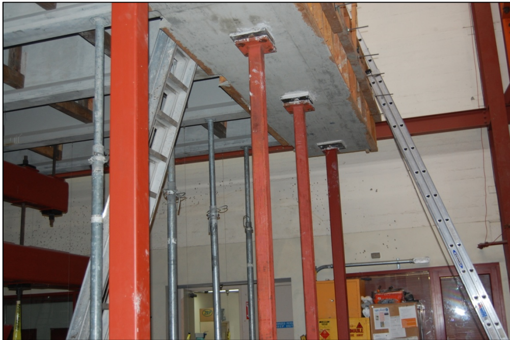
Figure 5.7: Temporary Support System Used Under Each Abutment
