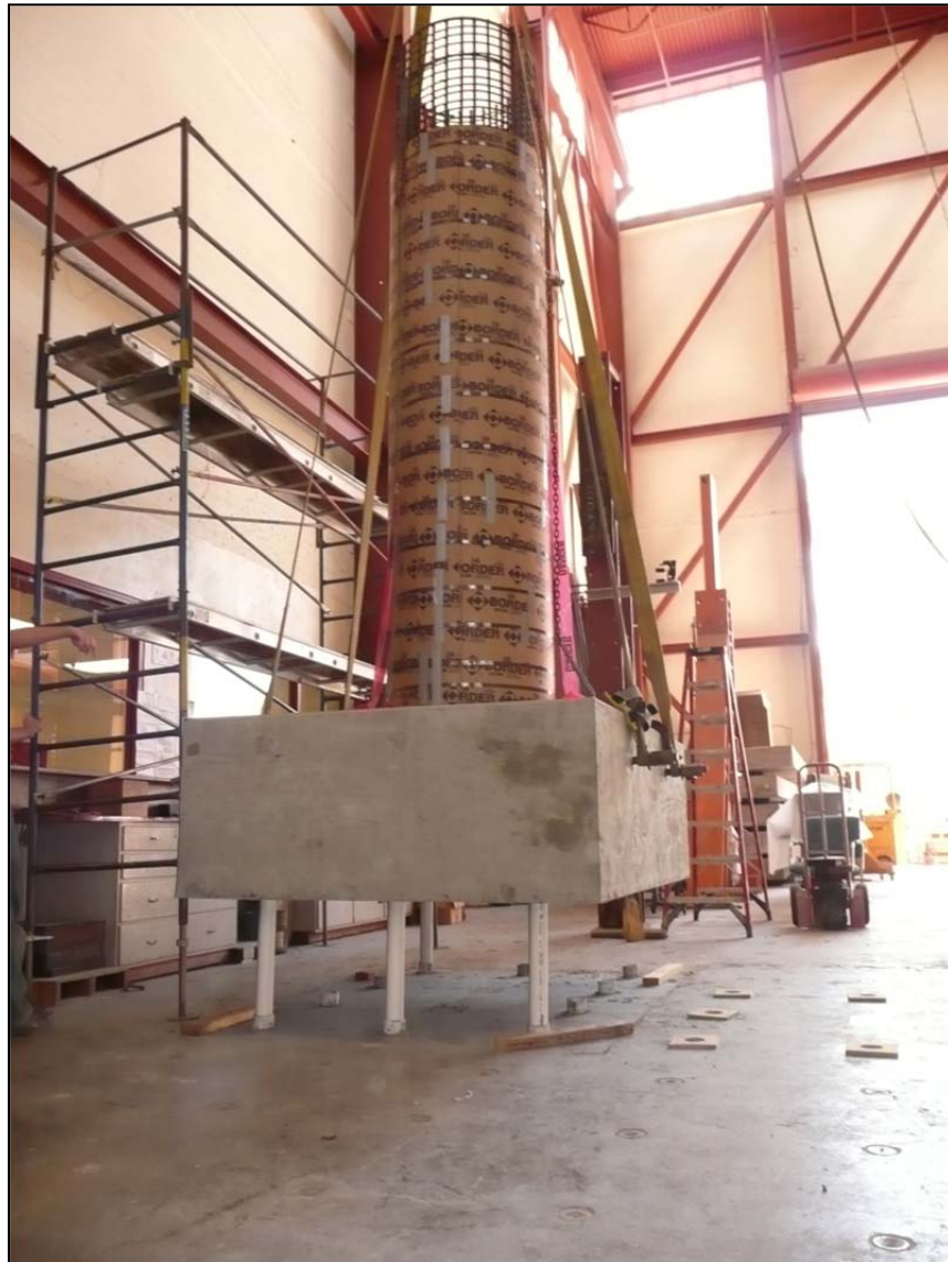
Figure 5.3: Repositioning the Column and Footing
