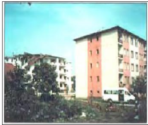
Figure 1.3 Precast concrete building that sustained no damage when subjected to the 1999 Kocaeli earthquake in Turkey (Ghosh, 2001).
