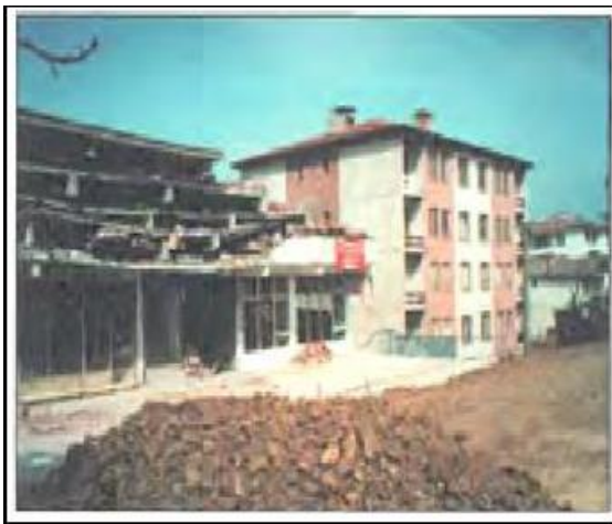
Figure 1.3 Precast concrete building that sustained no damage when subjected to the 1999 Kocaeli earthquake in Turkey (Ghosh, 2001).
