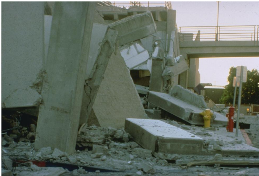
Figure 1.1 Collapse of the second level of the Northridge Fashion Center parking garage constructed using precast post-tensioned technology (Photo Credit: J. Dewey, USGS).
