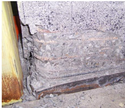
(c) Spalled region of wall in PreWEC-1
