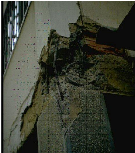
Figure 1.3 Joint Failure in the Cypress Gardens Building due to the Caracas Earthquake [3]
