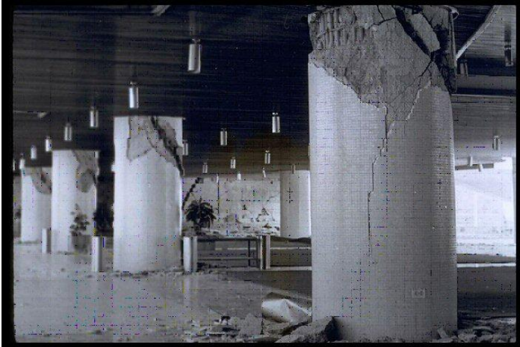
Figure 1.2 Damage to the 2 nd Story Columns of the Macuto Sheraton due to the Caracas Earthquake [2].
