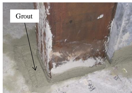
a) Pagel V 1A/40 grout at column-foundation interface
