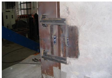
c) A view of an installed O-connector with restrainer near the base of the wall
