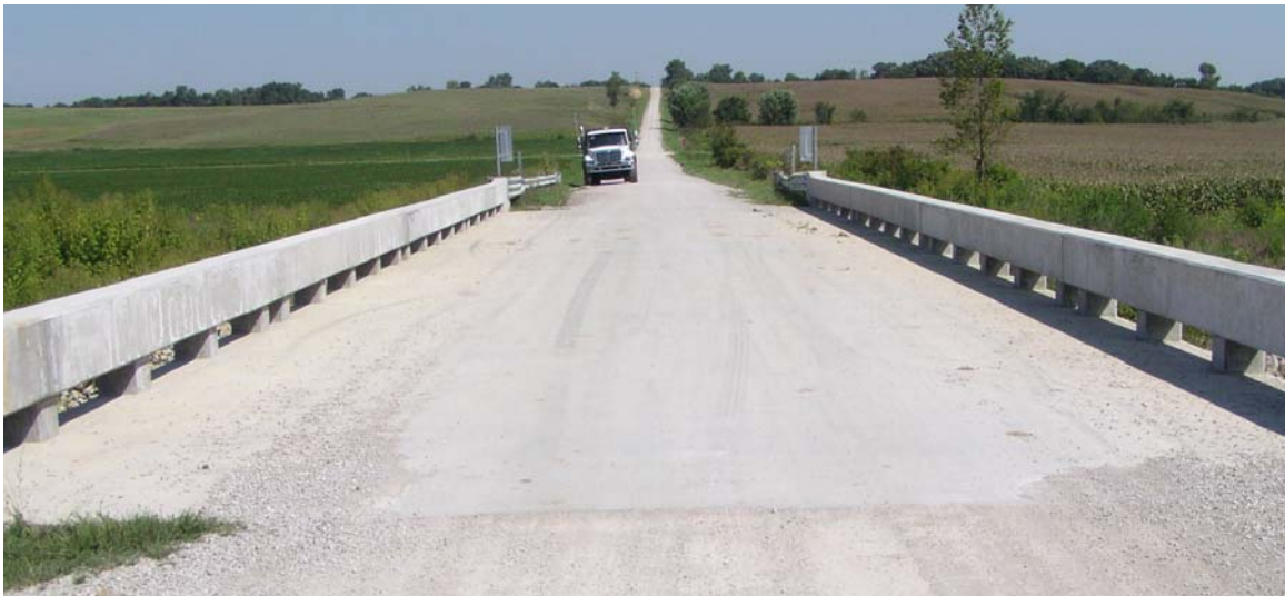
c) Tandem truck used during Test 1
