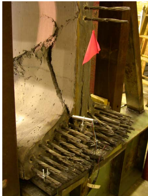
Figure 6.8. Vertical crack in web at west end of large-scale shear test beam after failure.
