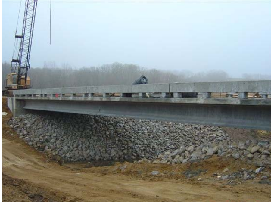
Figure 3.5. Elevation of Wapello County UHPC bridge.
